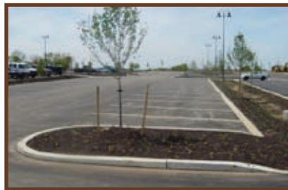
Top: Rain garden with overflow inlet in center of garden.
