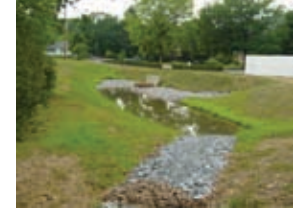
Infiltration beds collect runoff for on-site storage and infiltration.
