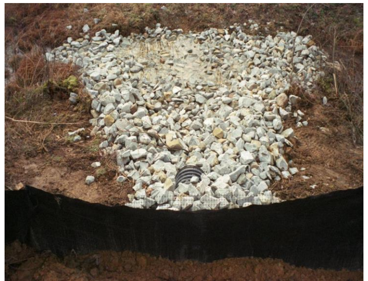
AN EXAMPLE OF ROCK OUTLET PROTECTION - From Erosion and Sediment Pollution Control Program Manual, PADEP, March 2012
