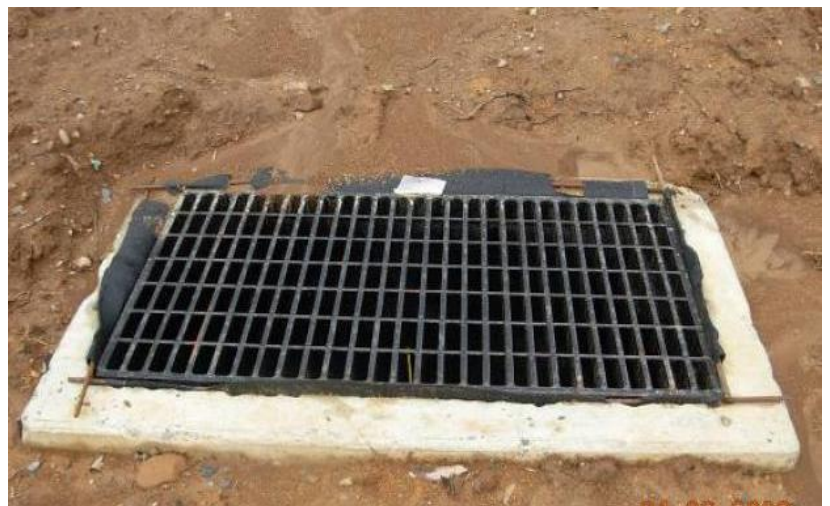
AN EXAMPLE OF AN INLET FILTER BAG - The edges of the bag can be seen around the grate. From Erosion and Sediment Pollution Control Program Manual, PADEP, March 2012 Courtesy Northampton County Conservation District
