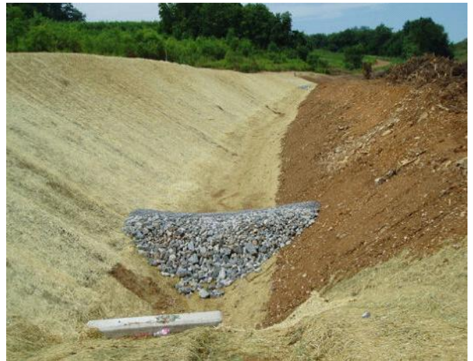
AN EXAMPLE OF A ROCK FILTER - Rock filters, such as the one above can be used to increase efficiency in swales. From Erosion and Sediment Pollution Control Program Manual, PADEP, March 2012 Courtesy of York County Conservation District
