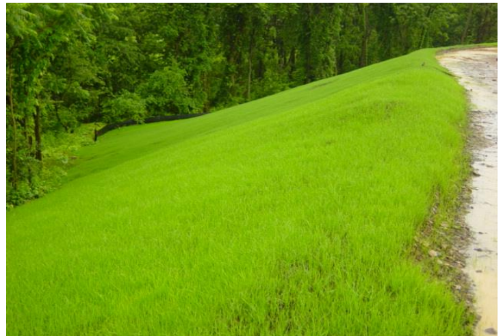
AN EXAMPLE OF VEGETATED STABILIZATION - Vegetation established on this slope prevents erosion. Courtesy of Dauphin County Conservation District
