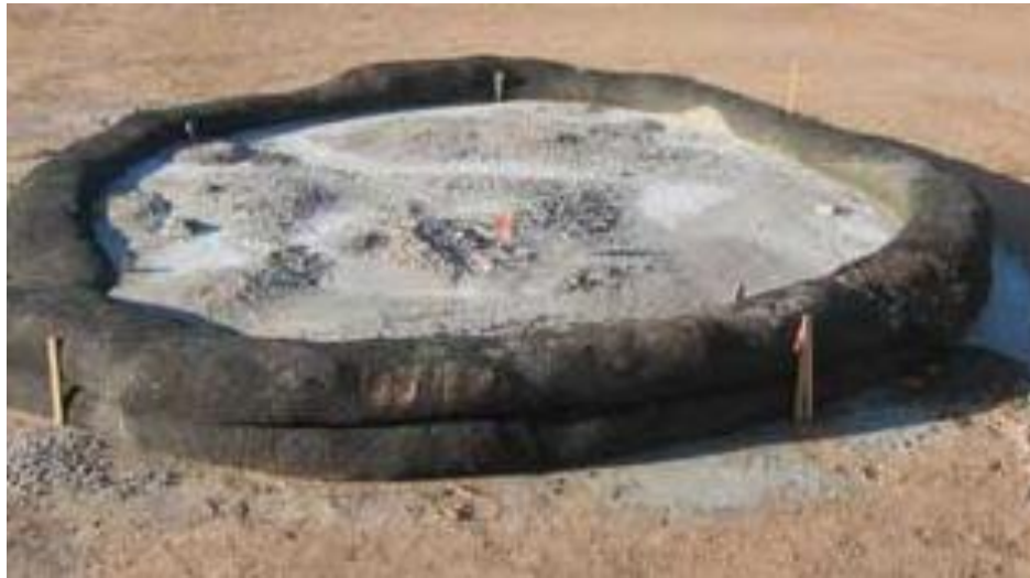
FIGURE 3.18 Typical Compost Sock Washout Installation
