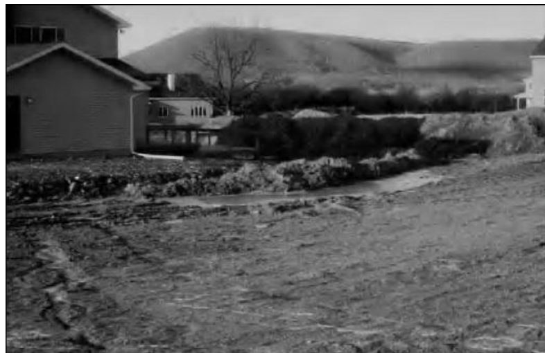
This soil's structure has been crushed and destroyed by compaction or mashed and destroyed by rough treatment.
