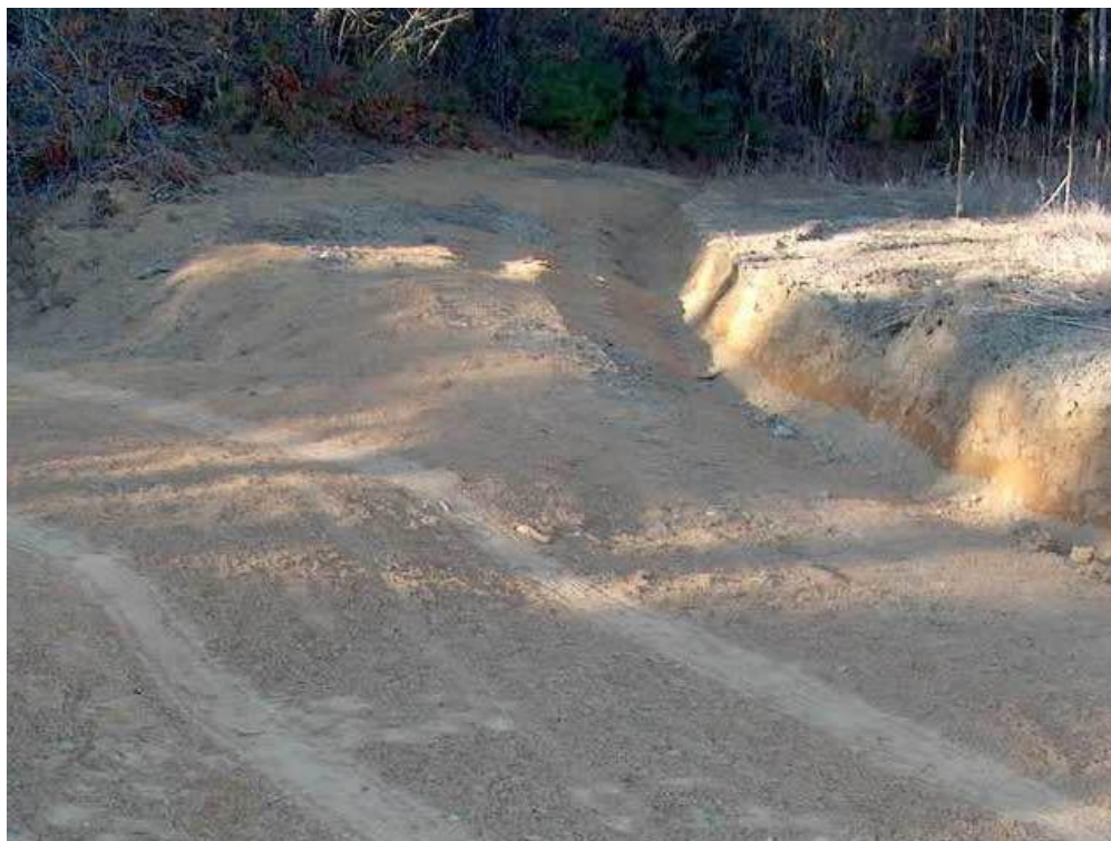
FIGURE 3.3 Typical Turnout
