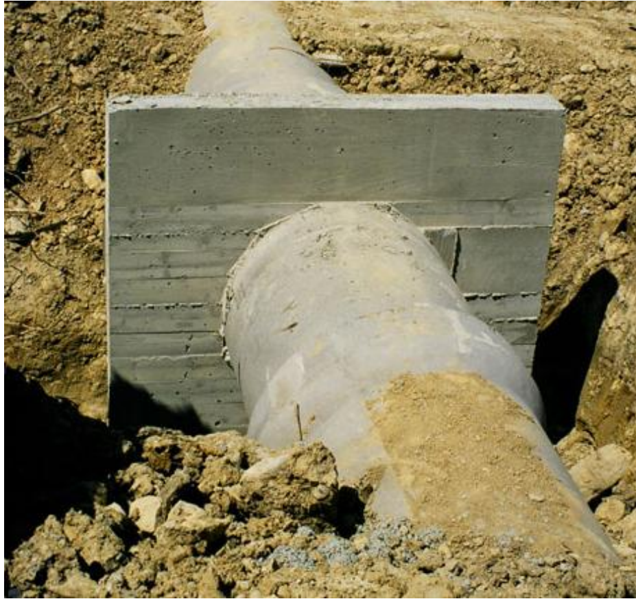
FIGURE 7.6 Anti-seep Collar Design
