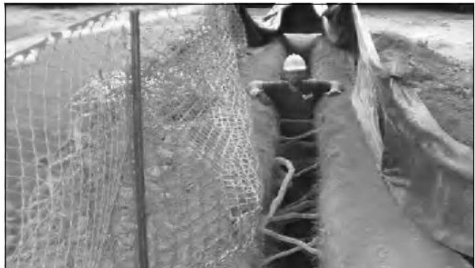
Air spades (radial trenching) can be used to break compaction under existing trees. Exposed roots must be protected from desiccation.
