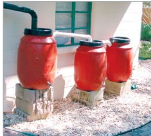
Multiple barrels provide for greater water storage.
