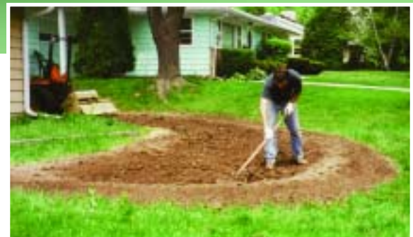
On a gentle slope, soil from digging out the garden can be used to create the berm. This rain garden is 4 inches deep.
