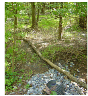
Basin at DCCD Tour Site #10
