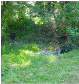
Basin at DCCD Tour Site #7
