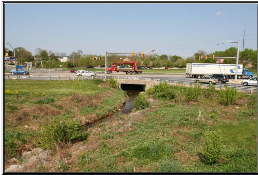
Photo 18 – Looking downstream at culvert under Hershey Park Drive
