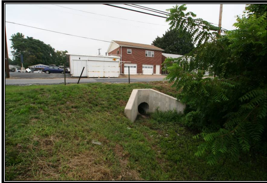
Photo 26 - Stormwater inlet under East Main Street
