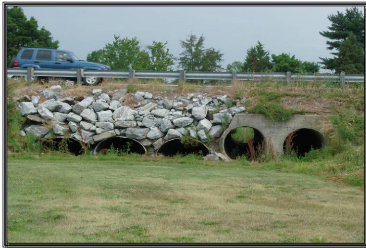
Photo 22 – Looking north at culverts under Route 422
