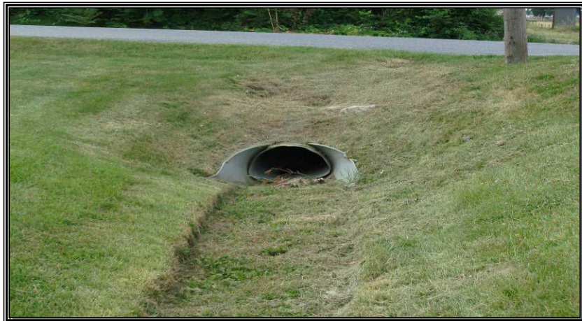
Photo 20 – Looking at the culvert under the driveway to Fudruckers Restaurant
