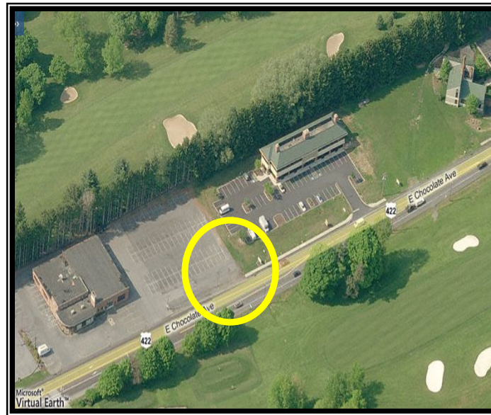
Photo 1 - Aerial View of Problem Area D1
