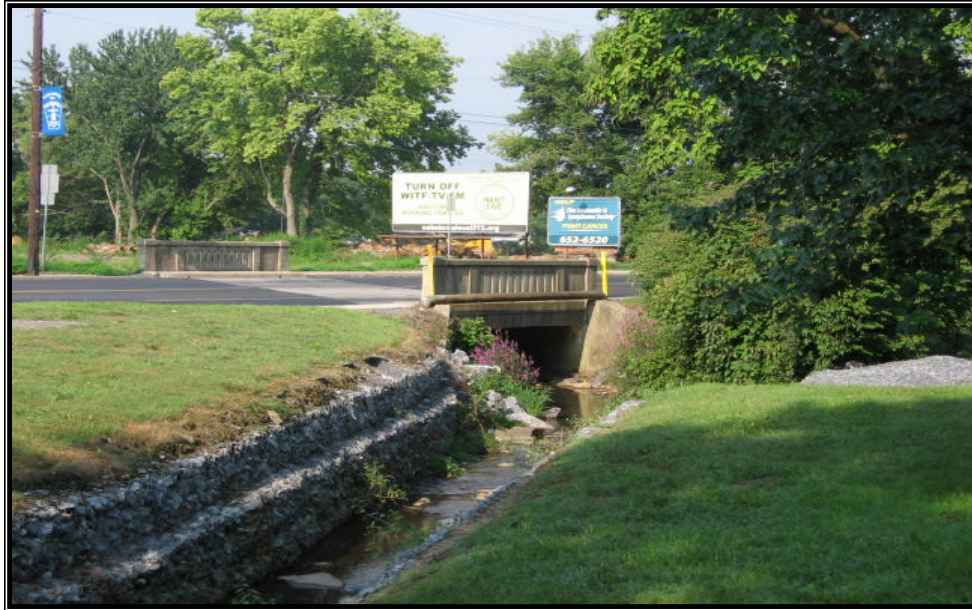
Photo 34 - Burd Run stream stabilization work
