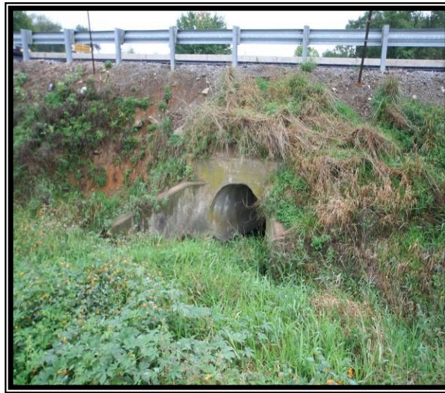
Photo 9 - Upstream end of the existing culvert under the Route 322 ramp
