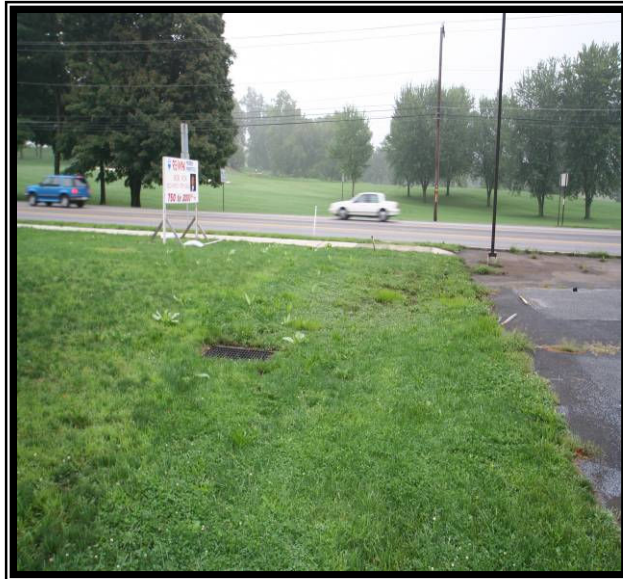
Photo 2 - View of the stormwater catch basin
