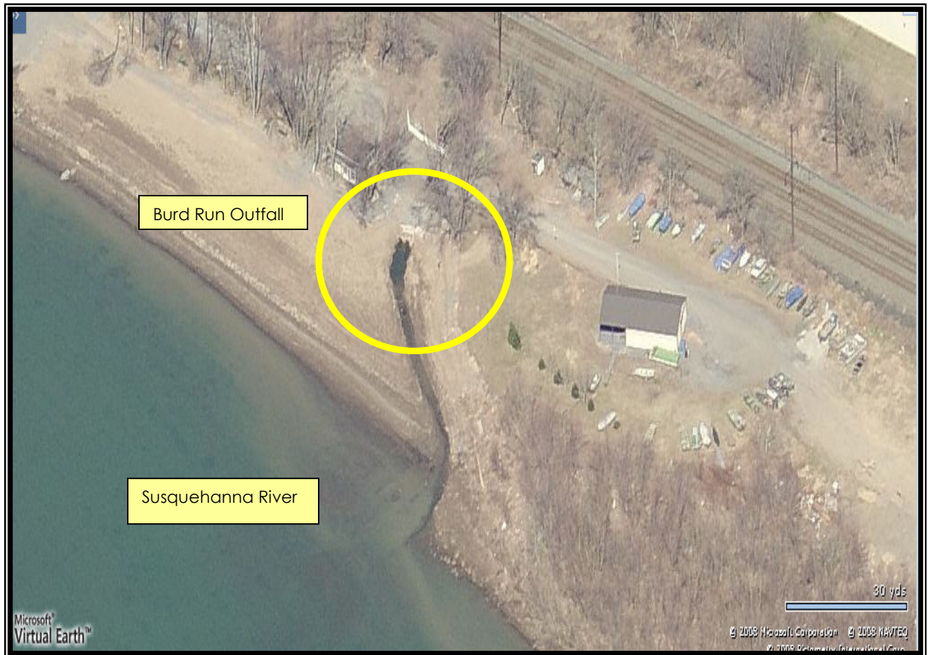
Photo 35 - Burd Run Watershed Outfall
