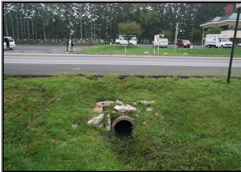
Photo 3 - Existing 18-inch pipe under Route 422
