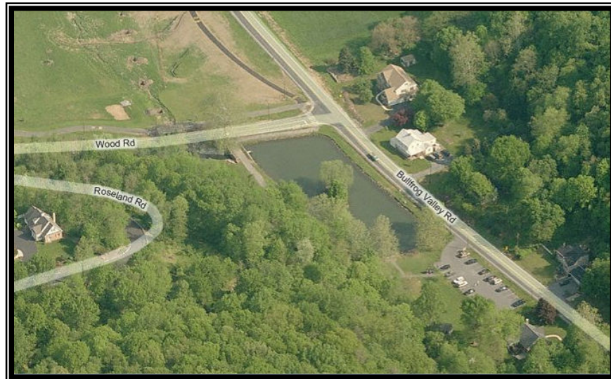
Photo 12: Aerial View of Wood Road
