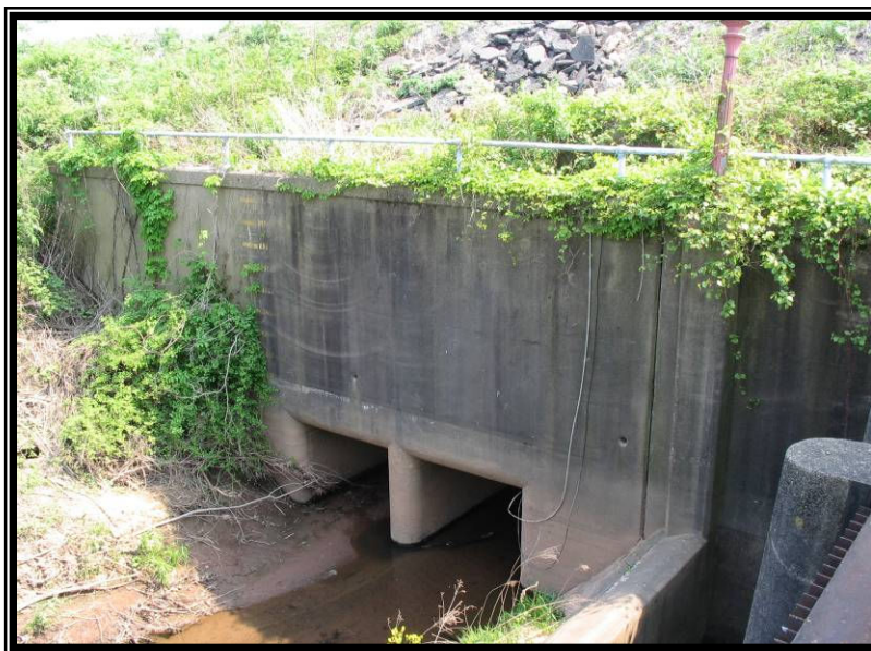
Photo 36 – Levee primary outlet culverts at HIA
