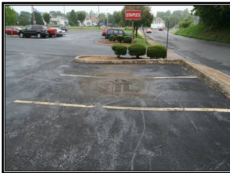
Photo 7 - Sedimentation and Flooding Problems at STAPLES
