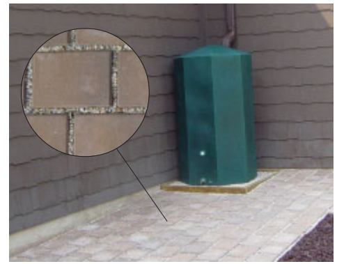
Block Pavers installed in Sitting Area
