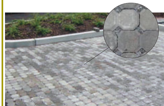
Block Pavers installed in Parking Area
