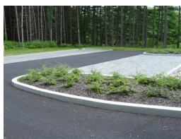
Porous Asphalt & Porous Block Paver Parking Area
