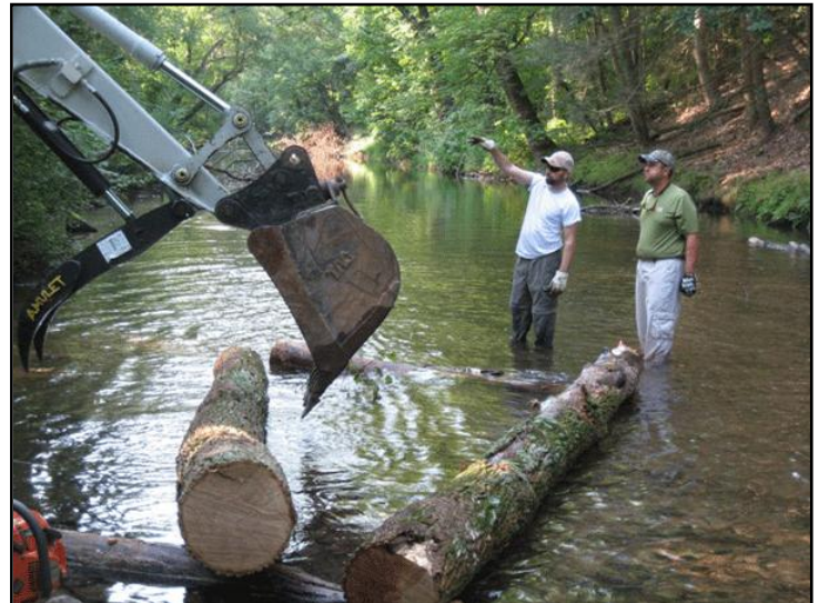
The Doc Fritchey Chapter of Trout Unlimited installing four log veins in Clarks Creek to protect streambanks and improve fish habitat
