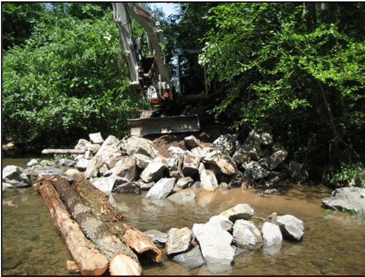
The Doc Fritchey Chapter of Trout Unlimited installing four log veins in Clarks Creek to protect streambanks and improve fish habitat
